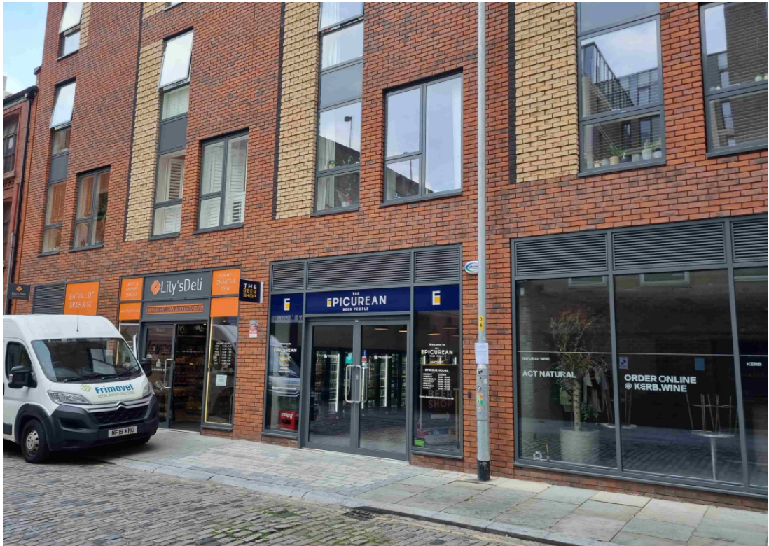
Neighbouring commercial units at the ground floor of Cotton House on the northern side of Henry Street located opposite the application site.
